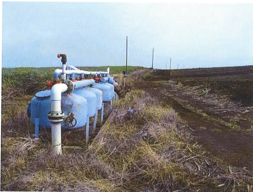
Photo No. 8: Dirt Access Road from Hamakuapoko Well No. 2 to Well No. 1 (East View)
