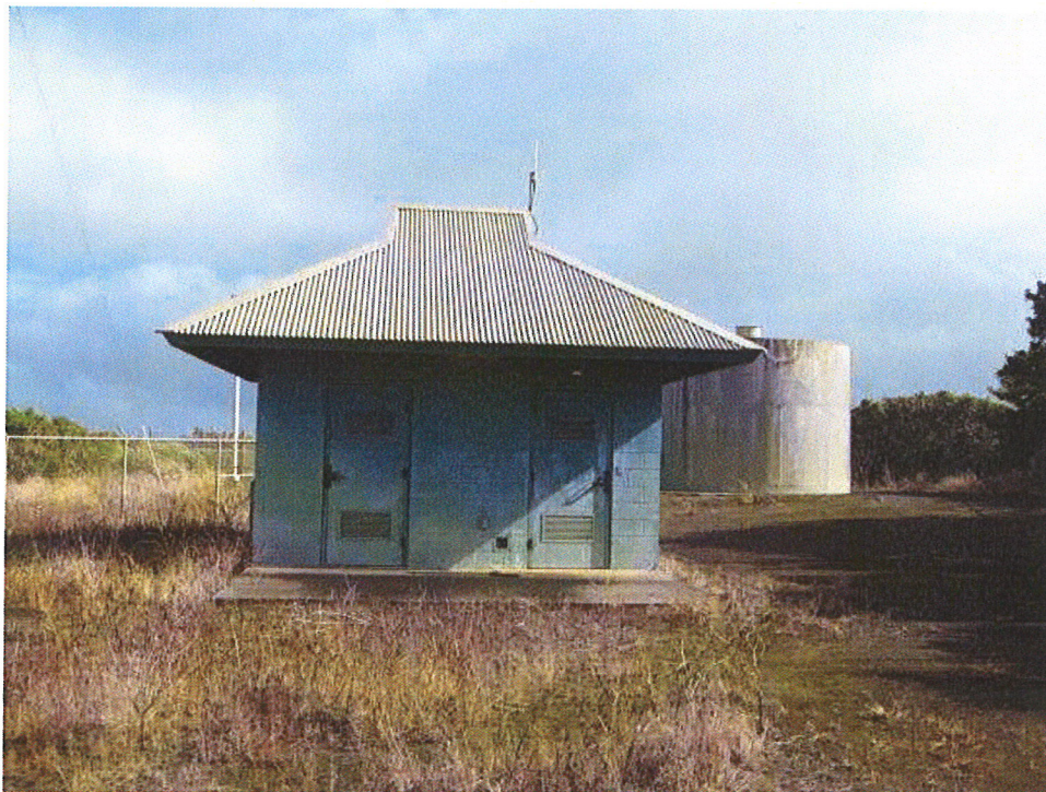
Photo No. 2: Hamakuapoko Well No. 1 Electrical Building (East View)
