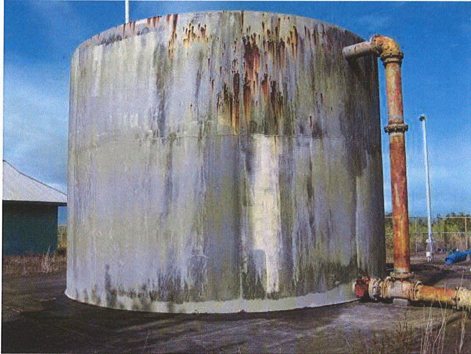
Photo No. 3: Hamakuapoko Well No. 1 Storage Tank (Northwest View)
