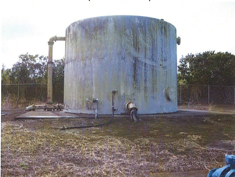
Photo No. 4: Hamakuapoko Well No. 1 Storage Tank (South View)
