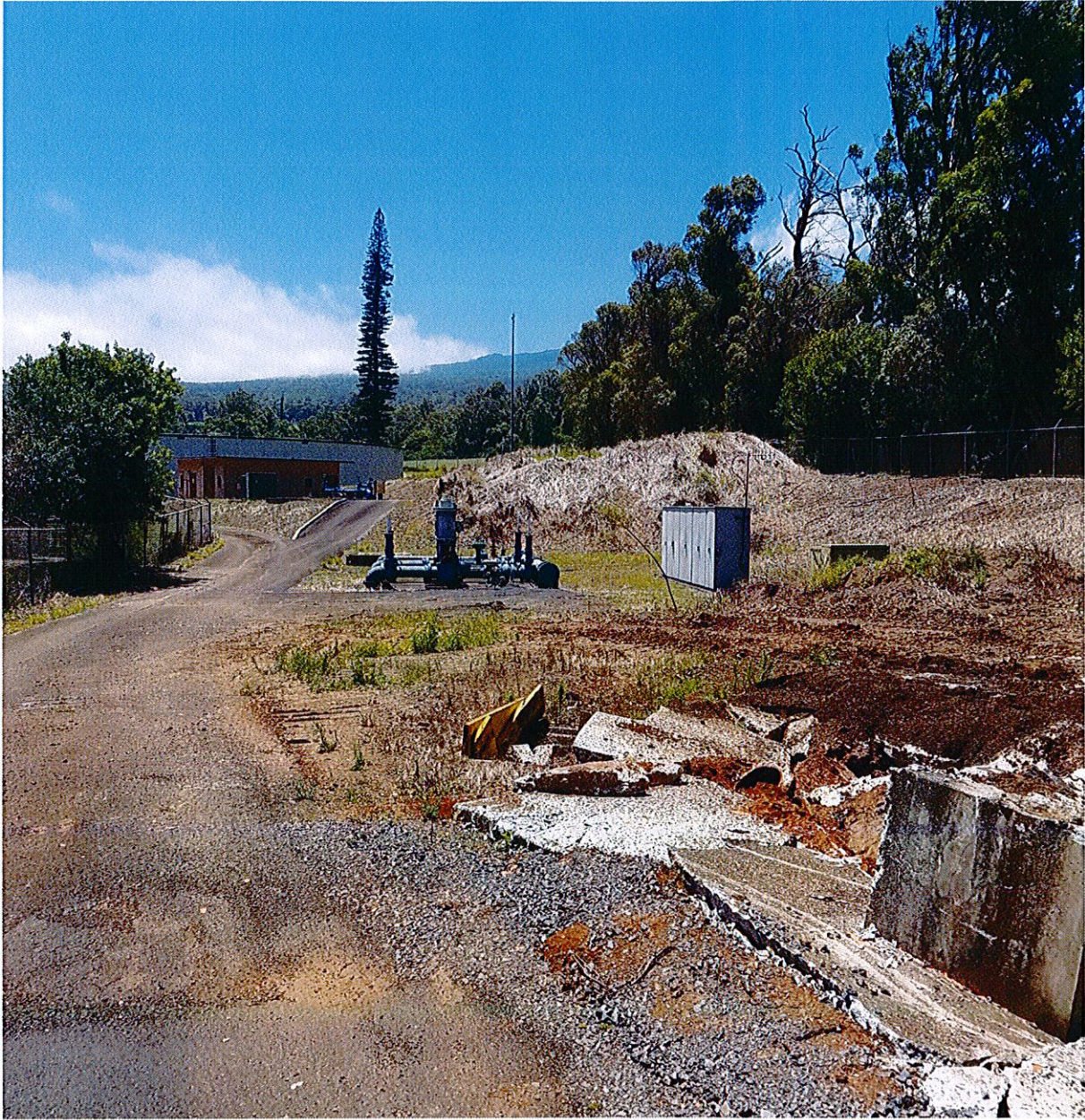
Figure 4: Central Portion of Project Area. View to East.
