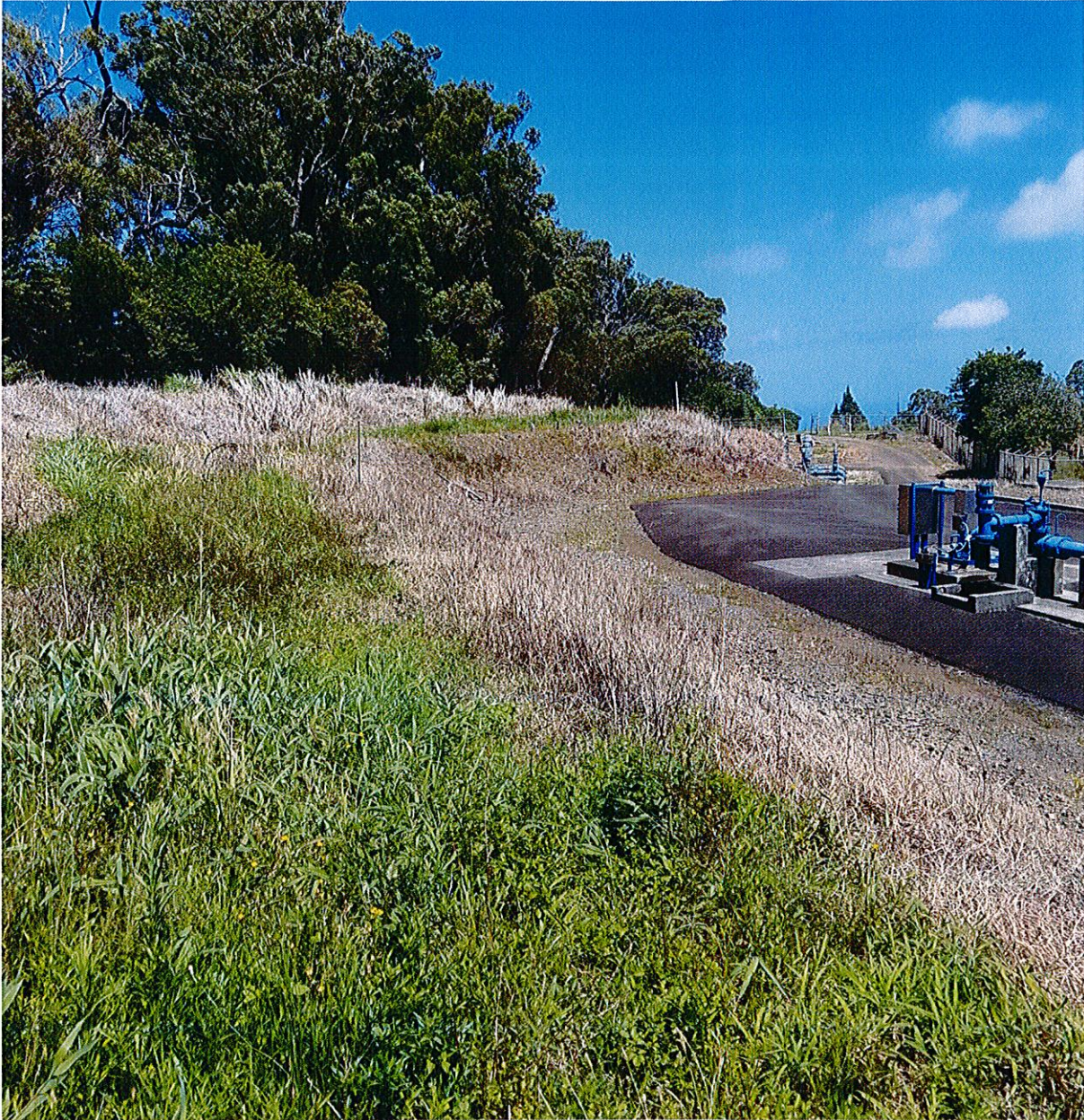
Figure 1: Northwest Flank of Project Area. View to Northeast.
