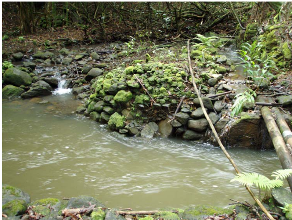
Note the two pipes on the right that pass over the ditch and transport water from stream. They are connected to one pvc pipe which empties back into the stream downstream.
