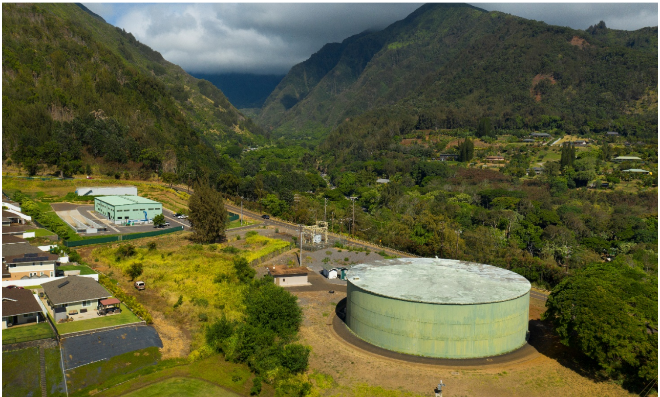
Aerial view of the Iao Water Treatment Facility. Photo courtesy of Shane Tegarden.
