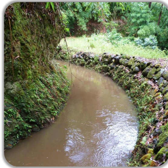
Center Ditch, stacked rocks on right wall and bedrock on left wall
