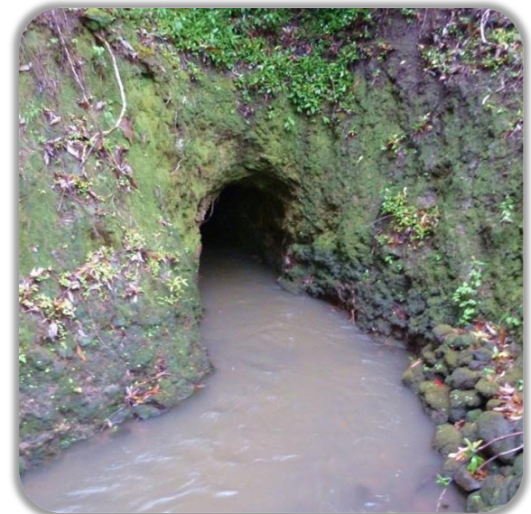
Manuel Luis Ditch, typical tunnel
