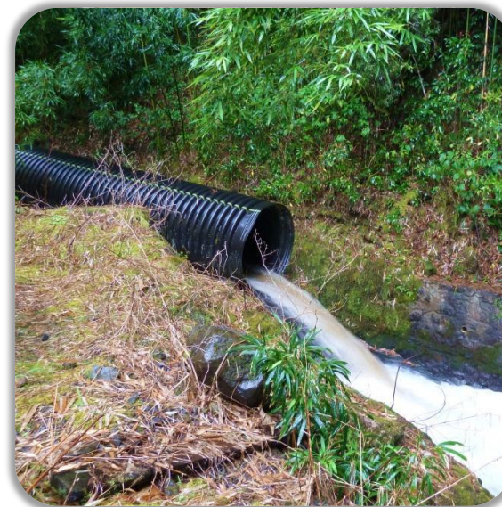
Lowrie Ditch, pipe section of the ditch
