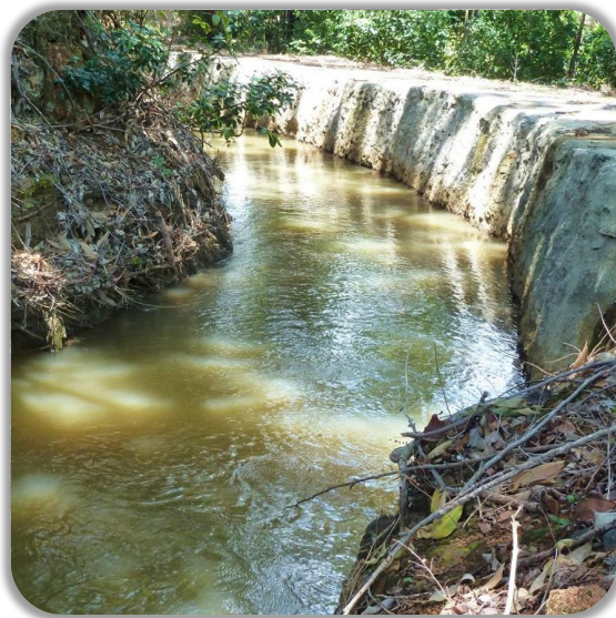
Lowrie Ditch, concrete on right wall (repaired) and earthen material on left wall
