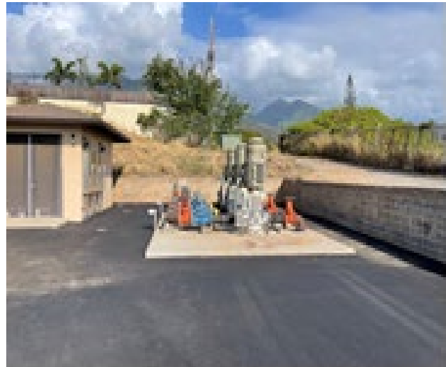
(Left:) Mokuhau installation of on-site generator that applies electricity to a solution of salt and water to produce sodium hypochlorite used for disinfection of well water. (Right:) Upgraded Waiale booster pump station.
