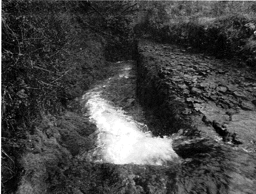
Figure 4-10. Photo shows water from the reservoir flowing into the ditch. (3/12/2009; Tributary name: Kōlea (64003001); PBN: sh004p-032-031209; Photo by: Hau, S.; SBN: sh004d-031208; Lat. (DD): 20.87175, Long. (DD): -156.18997).
