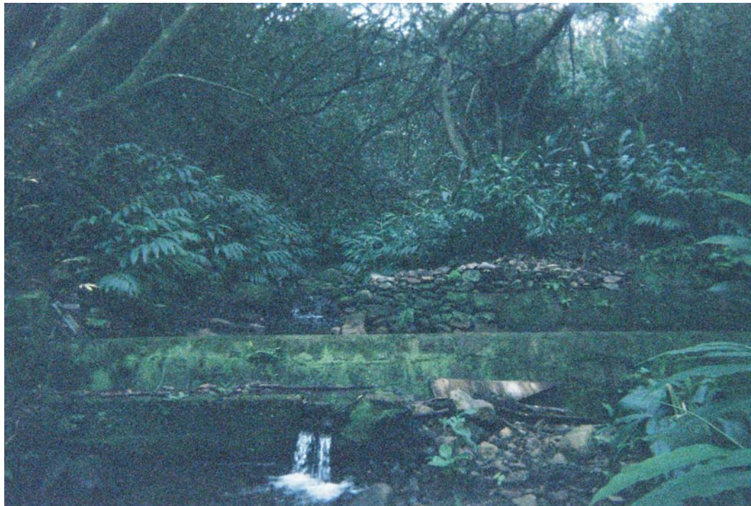
Water flowing from two pipes with diversion into Irrigation Ditch above diversion by Ernie Schupp taro patches (lo'i).
