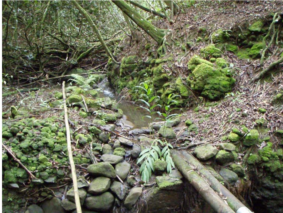
Water collection by two pipes over Lowrie Ditch.
