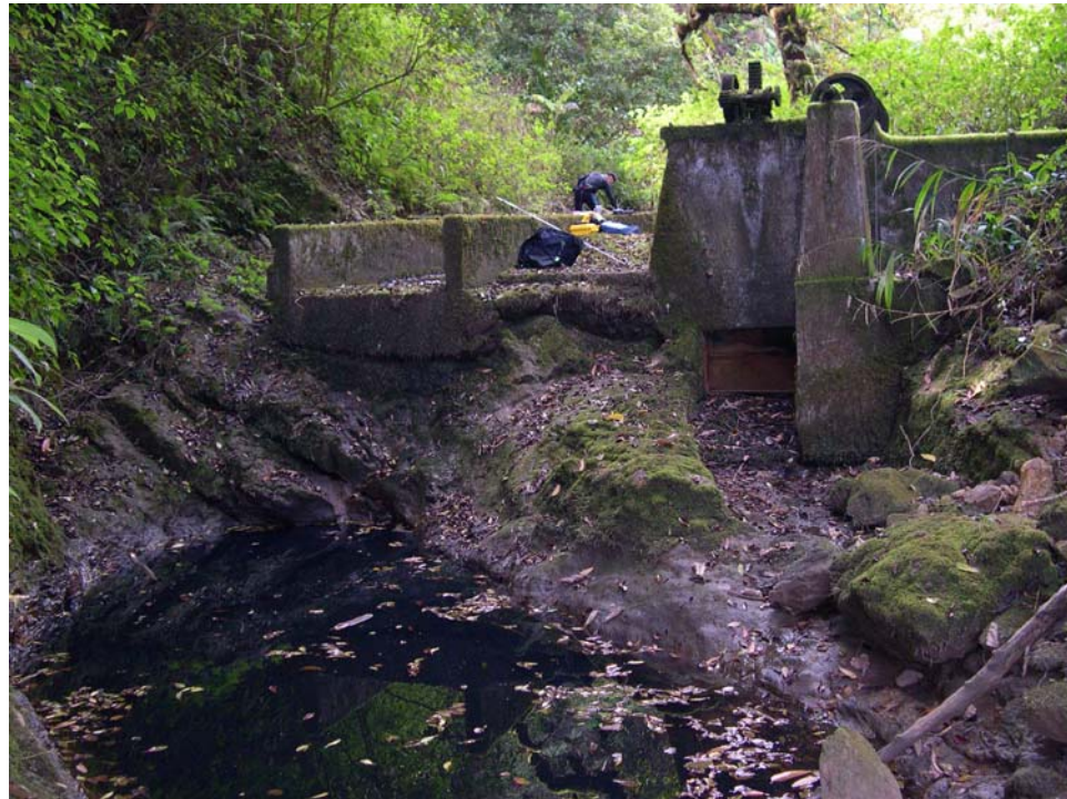
Upstream view of first diversion above jeep road at site gh003r-030408
