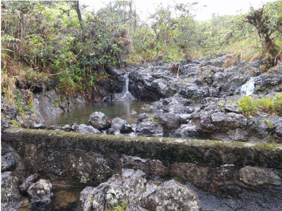
Figure 5-15. Photo shows a wall that diverts the water from the stream. (2/10/2009; Tributary name: Pa'akea (64019003); PBN: dk005p-024-021009; Surveyor: Kuamo'o, D.; SBN: dk005d-021009; Lat. (DD): 20.81321, Long. (DD): -156.11987).
