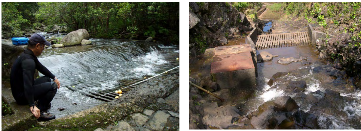
Figure 19. Stream diversion intakes on Waihe'e Stream (left) and Honopou Stream, Maui (right). Notice how 100% of the water flows into the diversion at this discharge. An animal moving downstream would be transported with the water and entrained in the diversion structure resulting in 100% mortality.
