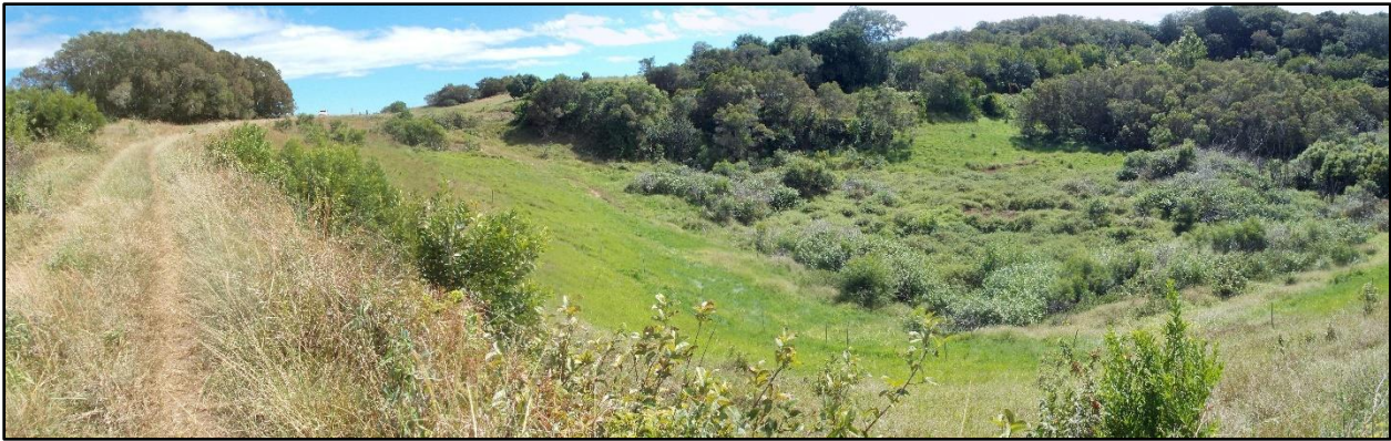
Figure 8. The reservoir basin with the dam crest vehicle pathway on the left. View facing southeast. MASON, 2023.
