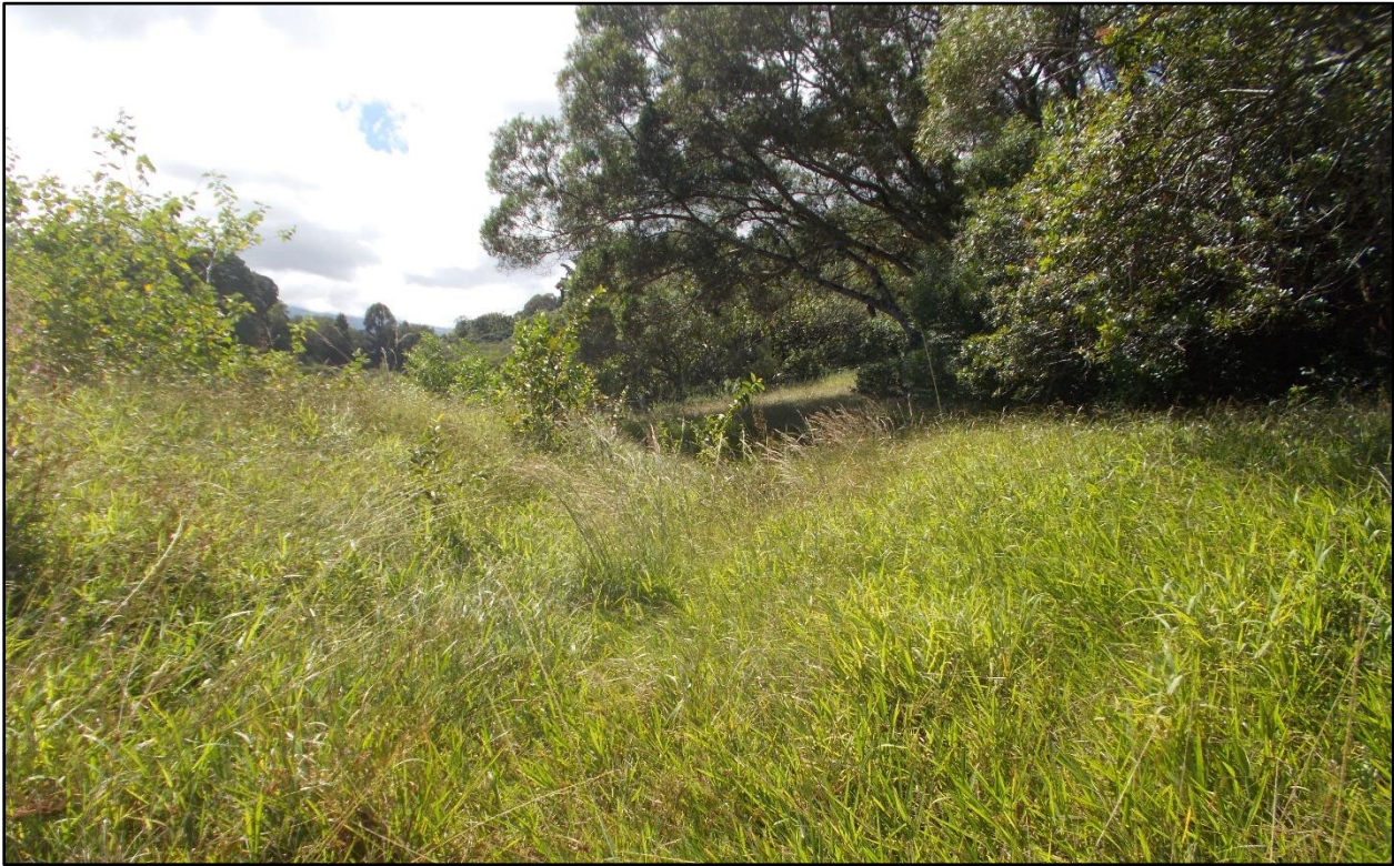
Figure 9. The dam spillway. Looking up the spillway toward the reservoir basin. View facing south. MASON, 2023.
