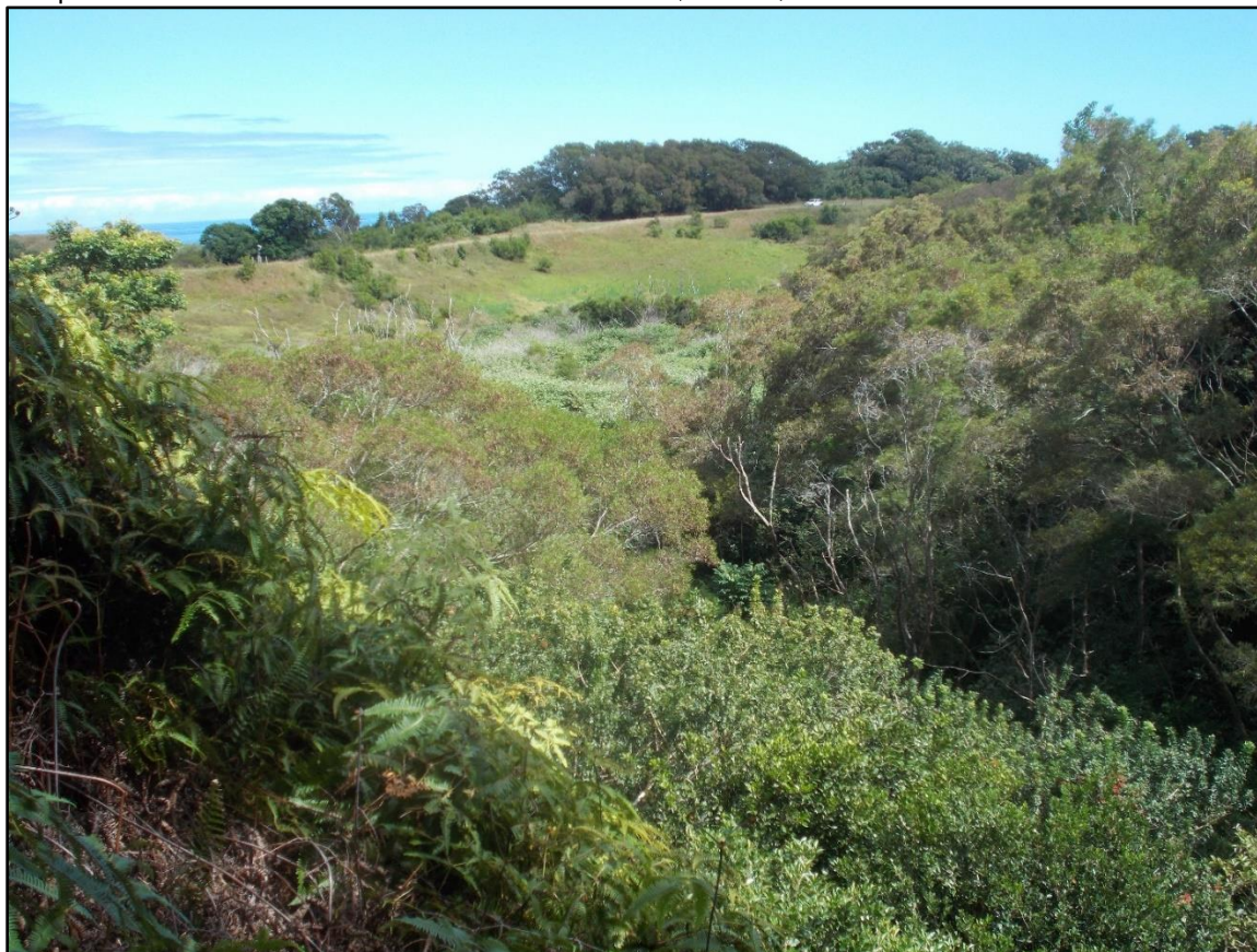
Figure 7. Kapala'alaea Reservoir basin, with the dam in the background. View facing north. MASON, 2023.
