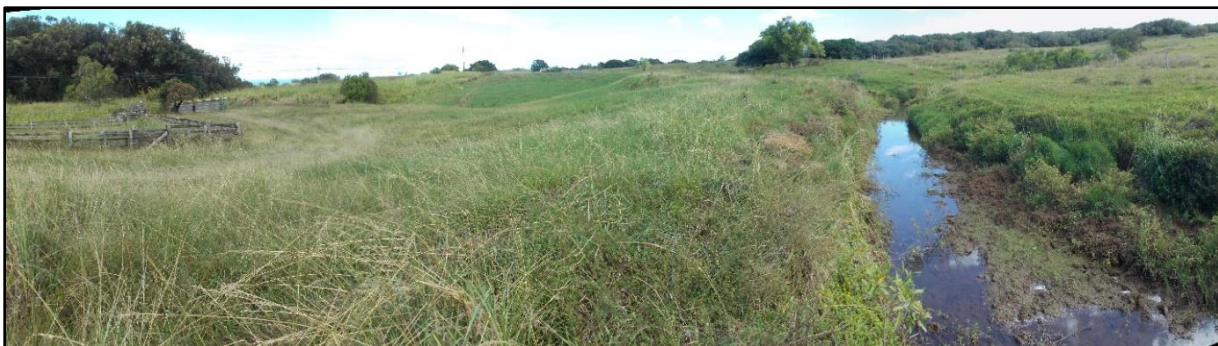
Figure 15. A typical section of ditch northeast of the Kapala'alaea Reservoir. This view shows the open land between the ditch and the highway, to the left. This area is proposed for depositing excavated dam material. View facing east. MASON, 2023.
