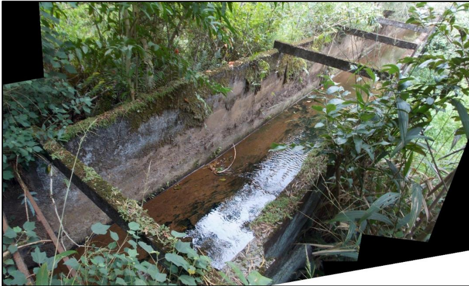
Figure 22. Concrete flume on the Lowrie Ditch. View facing southwest. MASON, 2023.
