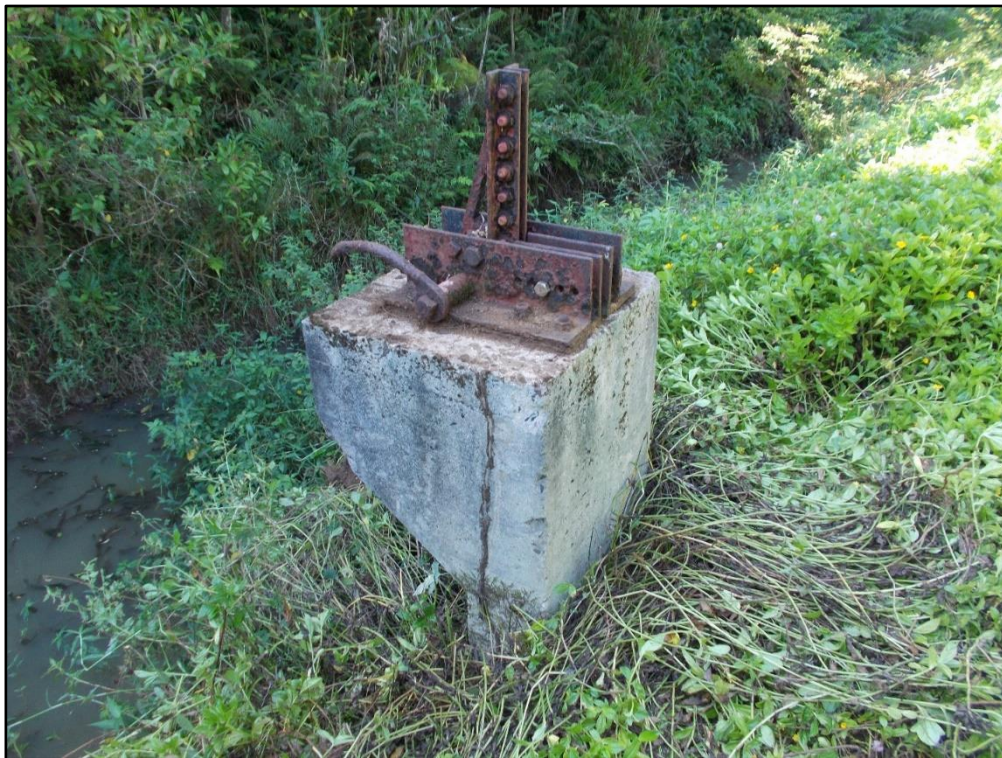
Figure 18. Ratchet Type gate that formerly functioned to sluice water from the Lowrie Ditch into the Kapala'alaea Reservoir. This gate is now fixed in the closed position. View facing south. MASON, 2023.
