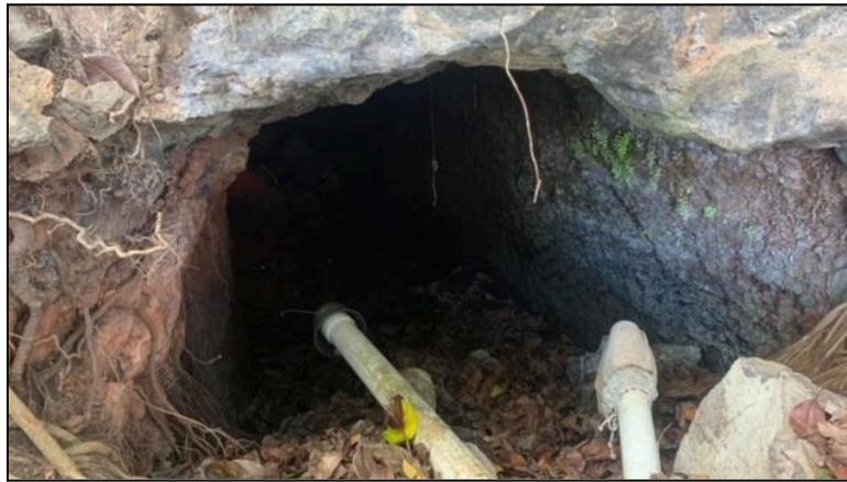
**Figure 25:** Man made spring created by drilling into a cliff face 12 meters above the property.
