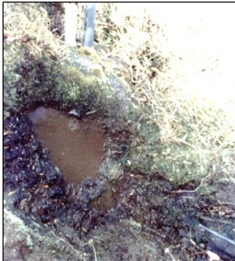
K-24c Intake at Ko'olau Ditch
