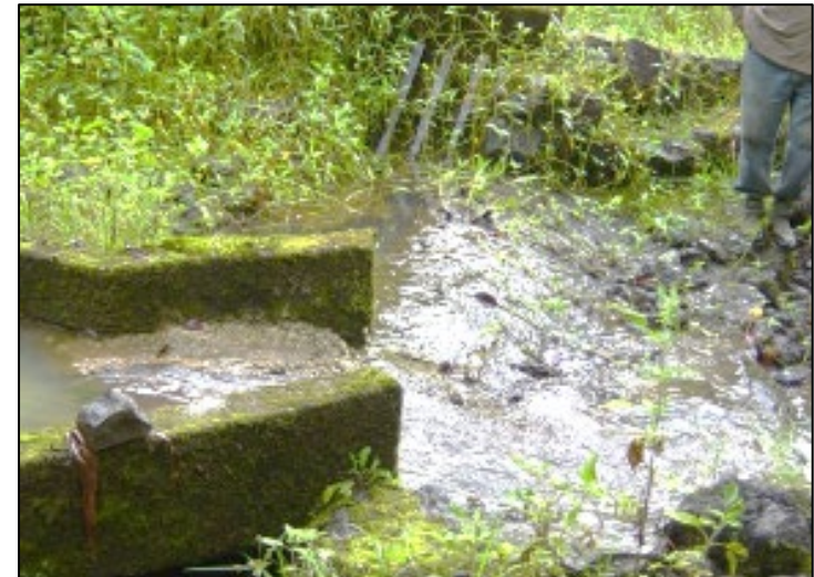
Kikokiko Small Intake at Ko'olau Ditch
