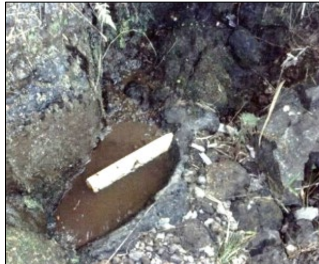
K-24e Intake at Ko'olau Ditch
